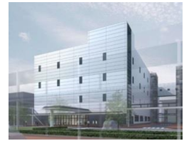
Exterior image of new manufacturing equipment
